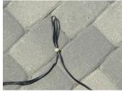
keep it from being damaged when digging in the yard and so it can be easily located. Form a loop in the cable where the lights will be located (with a rubber band if desired) to leave enough slack for connection of the light to the power cable.
