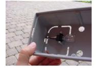
6. Run the low voltage cable which will supply power to the lights around the perimeter of your project. For installation with segmental pavers, you may set the cable atop the bedding sand under the border course of pavers to
