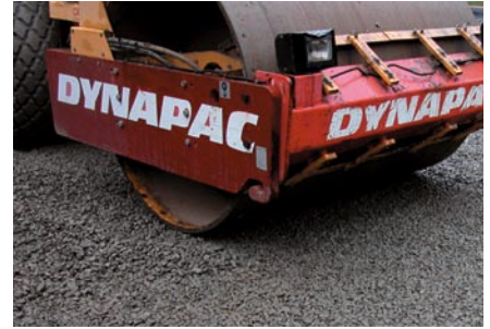
3. Compaction of the lower sub-base.
