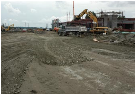
1. Excavation of sub-grade, removing any organic material.
