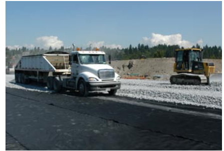
3. Clear crushed open-graded aggregate lower sub-base is placed, followed by grading and compaction.
