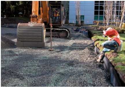
4. Placing and spreading the clear crushed open-graded upper sub-base.
