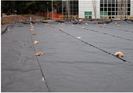
1. Placing the AP-SC1000 or 2000 woven geotextile with the specified overlap.
