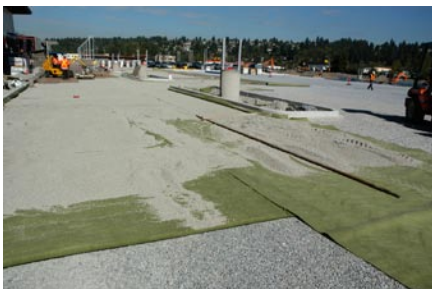
7. SC Inbitex® is placed followed by the 5mm clear crushed open-graded bedding course .
