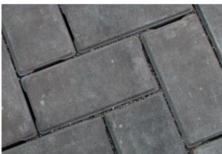
13. Close-up view of the joints with AP Engineered Joint Stabilizer applied before final compactions.
