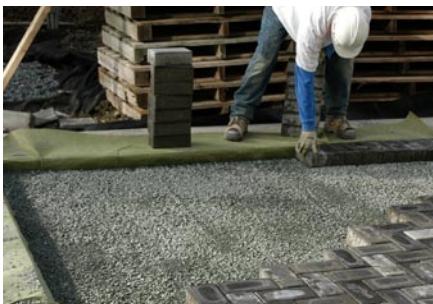
10. Placing the AquaPave® pavers.
