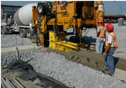
4. Paver restraints are placed.
