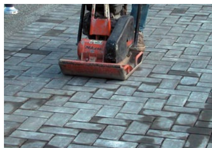
14. Final compactions of the AquaPave® pavers.
