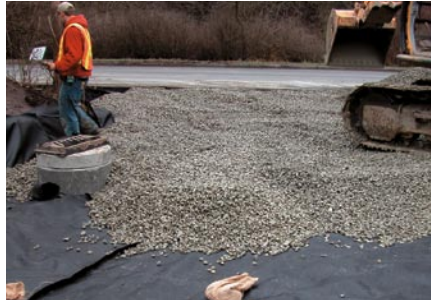
2. Placing and spreading of the clear crushed open-graded lower sub-base aggregate without wrinkling or folding the geotextile.
